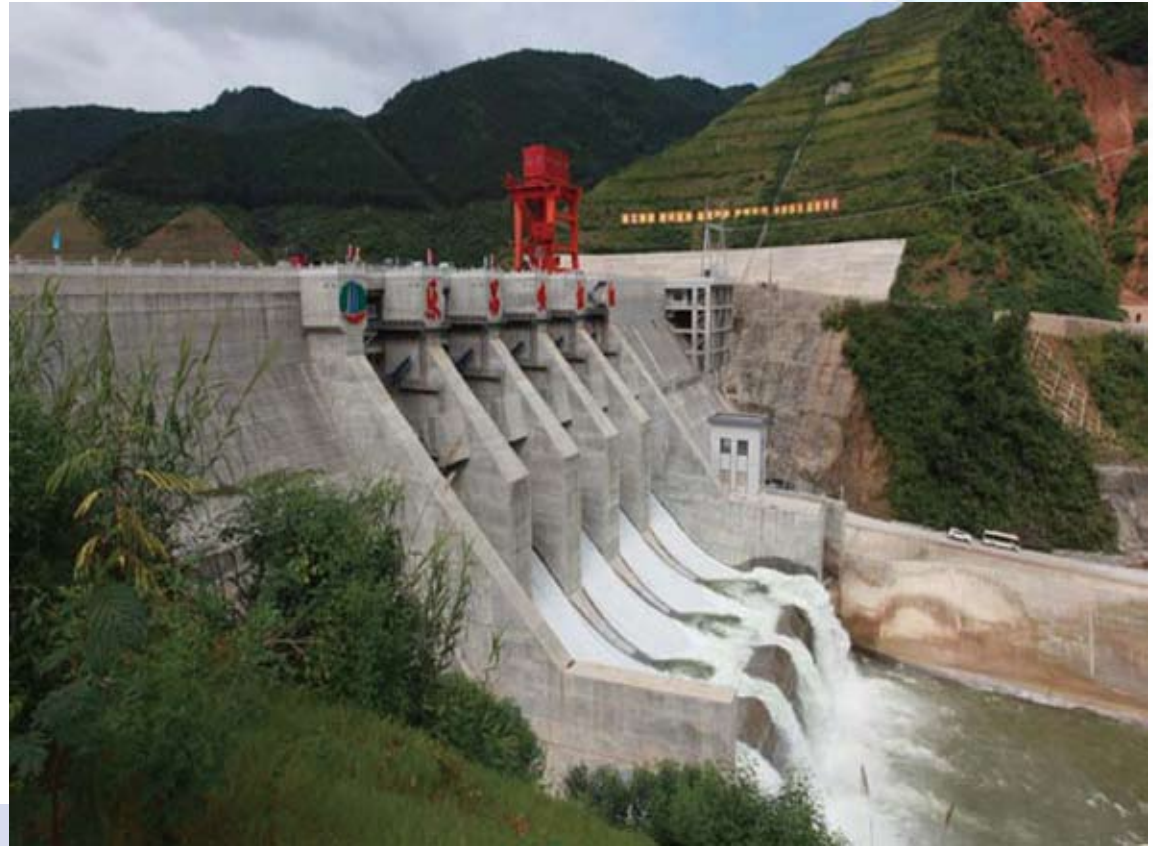
• 乐昌峡水利枢纽大坝安全监测自动化系统 Lechang gorge water conservancy dam safety monitoring automation system
