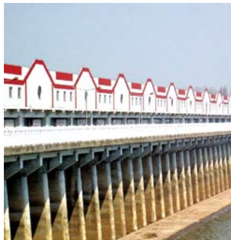
• 63孔闸门的大型水闸三河闸外景 63 large hole gate sluice cohesive material on location
