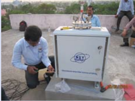
• 印度水情站设备安装 Hydrologic station equipment installation, India
