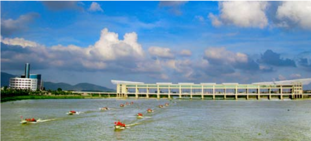
• 泉州金鸡拦河闸自动控制系统 Quanzhou golden block penstock automatic control system
